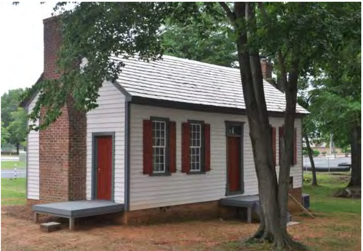
Northeast quarter facing interior of lot.
