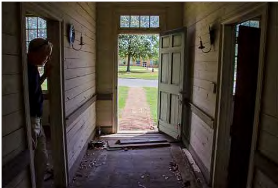
Central hallway looking south during restoration.
