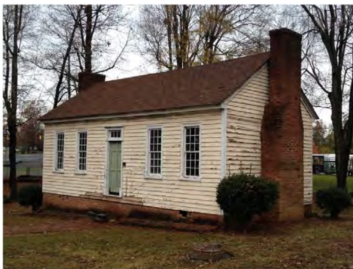
The 1976 restoration after a period of deterioration.
