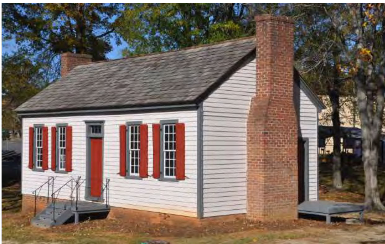
Southeast quarter facing Walker Avenue.
