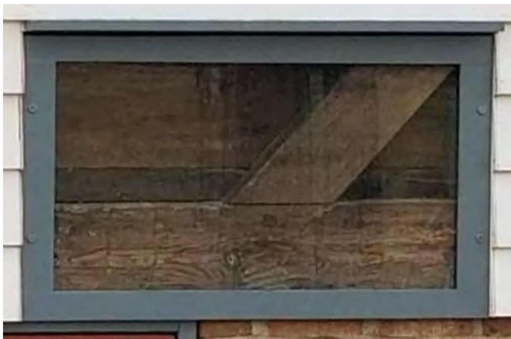
View window showing post-and-beam construction detail
